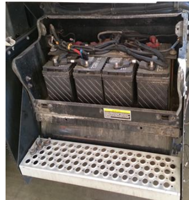
Figure 1: Existing Group 31 Lead-Acid batteries
