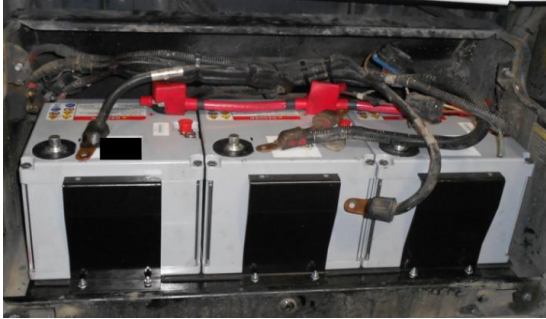
Figure 2: 6T batteries in the existing compartment
